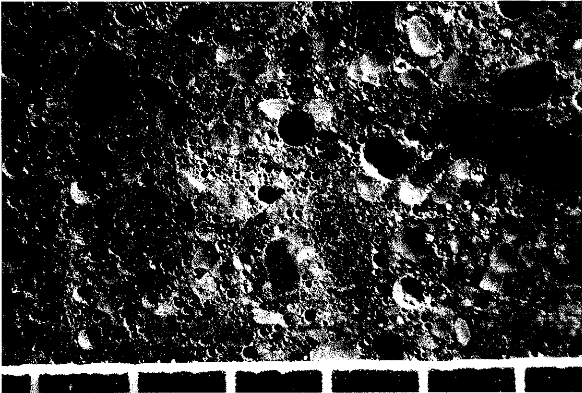
Figure 6 – View of the air void system in Core 1. Small areas with numerous voids that give the paste the texture of froth are visible (black arrow) as are the white secondary deposits of ettringite. Increments of the blue scale at the bottom of the image are \frac{1}{16} inch.
